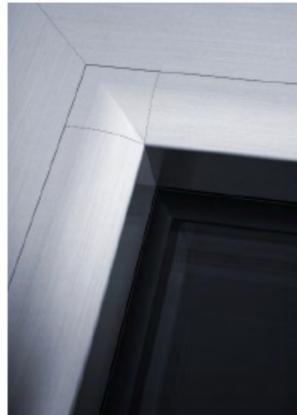
倒角玻璃扣條 Glazing bead with corner piece
